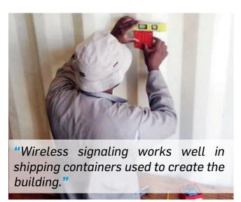
EMS donated all of the FireCell equipment to the system. This meant that with a little bit of extra funding from G2, the entire container house was fitted with a full EMS wireless system including fire control panel, optical smoke and heat detection, manual call points and sounders. The entire installation was completed in less than eight hours, including testing and commissioning.
