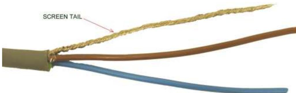
Figure 27 Power cable Screen Tail.
